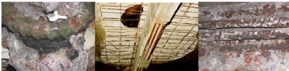
Corrosion Epoxy Coated Steel
